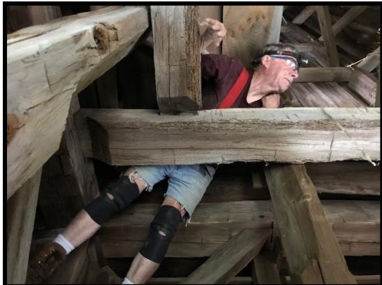
*Here is the steeple ...* In 2020 A hatch door blew off the steeple, dropping to the ground below. Church neighbors alerted us. Steve Woodard and Tom Hankinson climbed inside to do repairs ... Steve in the rafters; Tom behind the camera. The pair nailed in an ad hoc ladder with boards found in situ, then got the job done with tools winched up from below.
